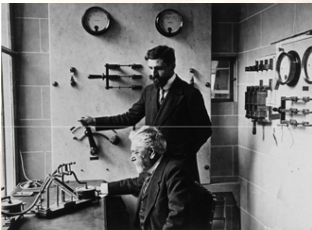
Eiffel and Lapresle in the control room, [4]
